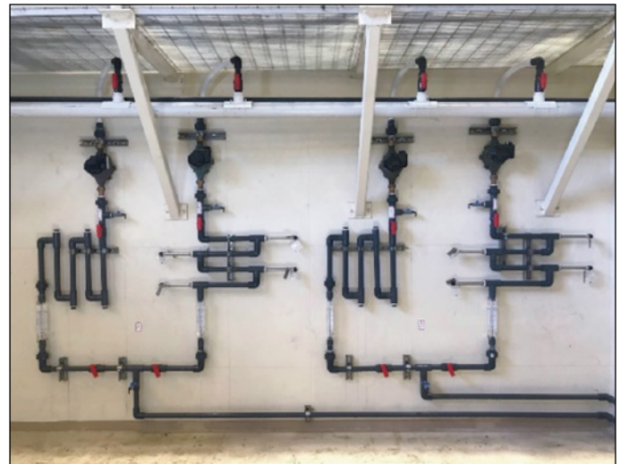
Figure 1: Corrosion test racks at the City of Sarasota.
